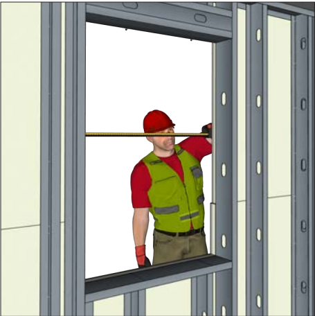
Measure the width of the punched opening.
