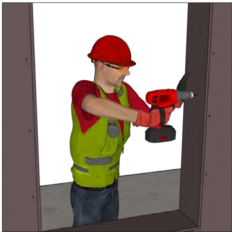
Install the side returns, following the Return Fastening Pattern .
