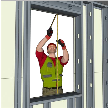
Measure the height of the punched opening.
