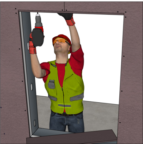
Follow the Return Fastening Pattern , above, install the top return.
