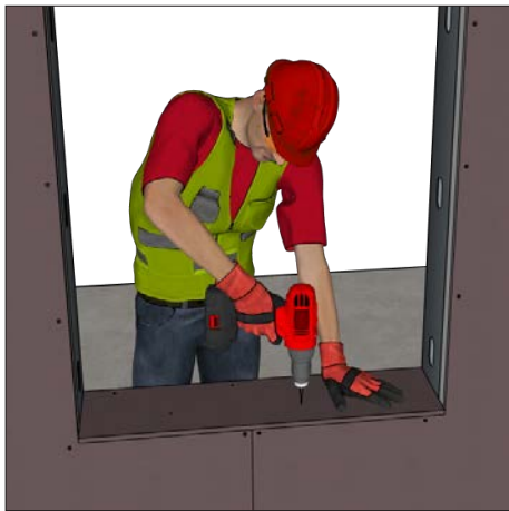
Install the bottom return, following the Return Fastening Pattern .
